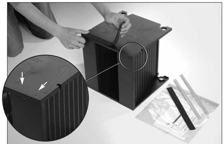
Step 2: Locate the gasket on the leaving air side of the half-cassette along the edge of the cassette side plate. A gasket location guide has been formed into the side plate. The gasket should be located to the outside of this line.
